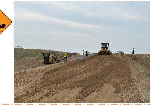
**Road Surface Conditions** Asphalt surfacing has been removed. Millings and aggregate base are being maintained for traffic.
